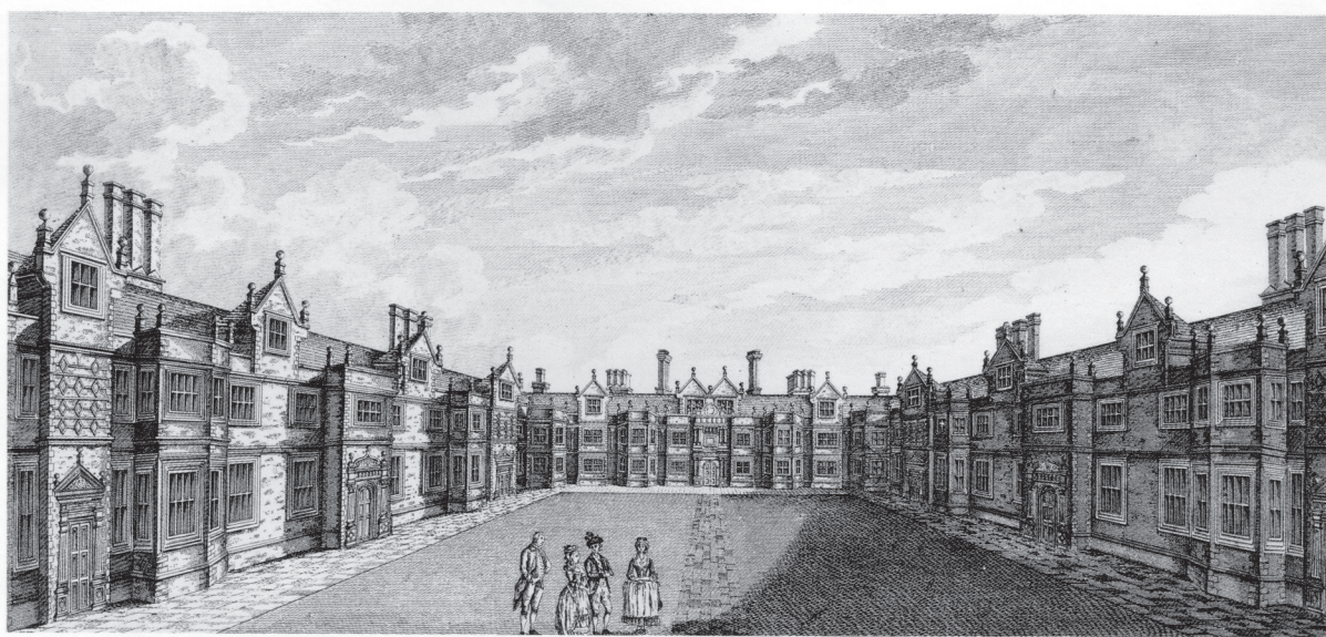
The Courtyard of the Elizabethan house. All but the top right-hand corner (the South Cottage) was demolished c. 1800
